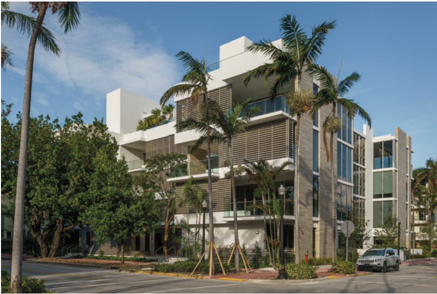
Louver House, Miami USA
